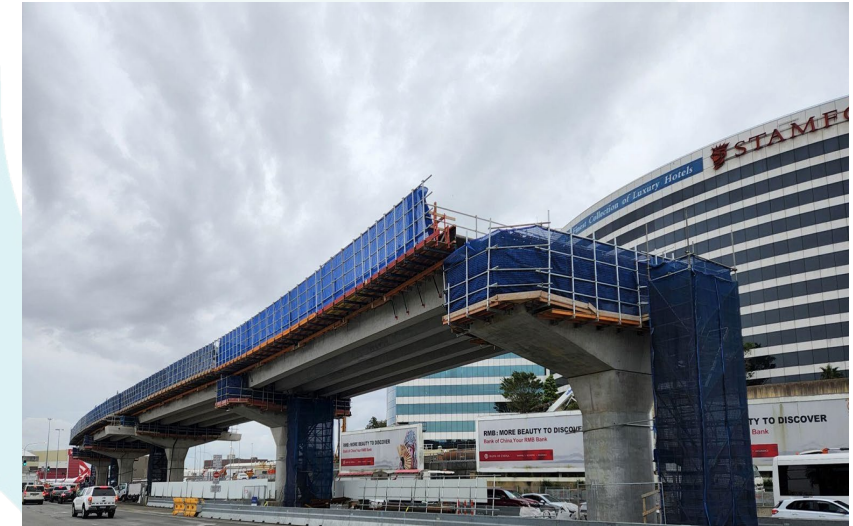
Case Study of Overpass Construction at the Gateway Project in Sydney
