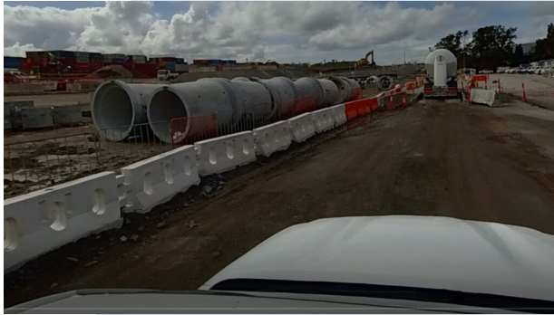
On-site Storage Yard of Precast Concrete Pipes and Raw Scan Data
