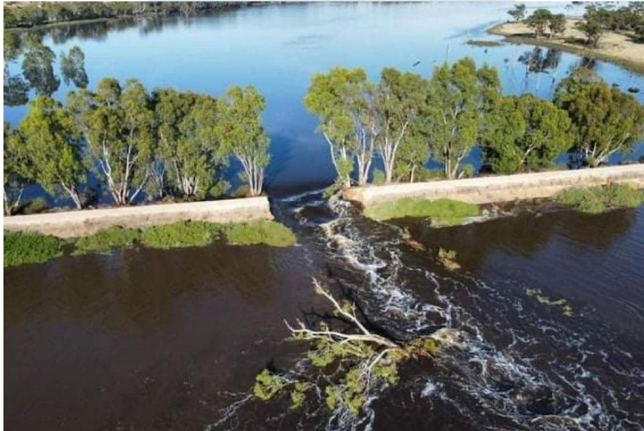
Failure of 50 levee banks along the River Murray, SA 2022.
